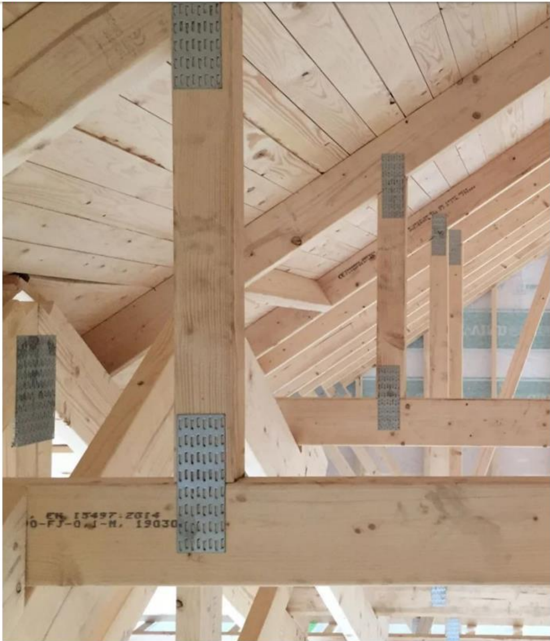
Roof trusses in construction timber.
